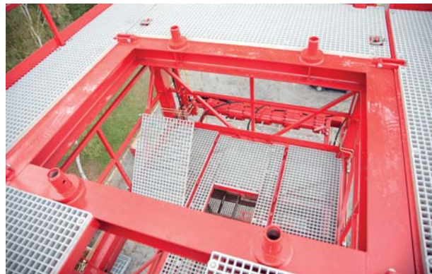
Injector platform with centering bolts
